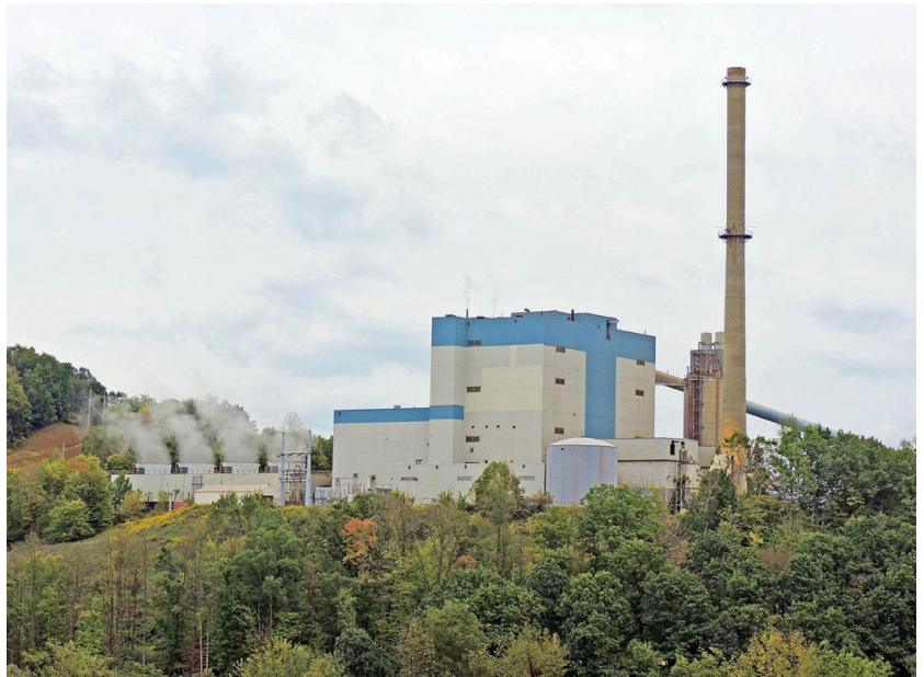
Grant Town Power Plant,
